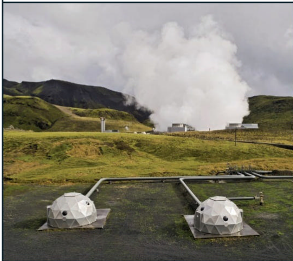
A Climeworks site in Iceland. Captured CO 2 is mixed with water and pumped underground, where it reacts with basalt rock and solidifies
